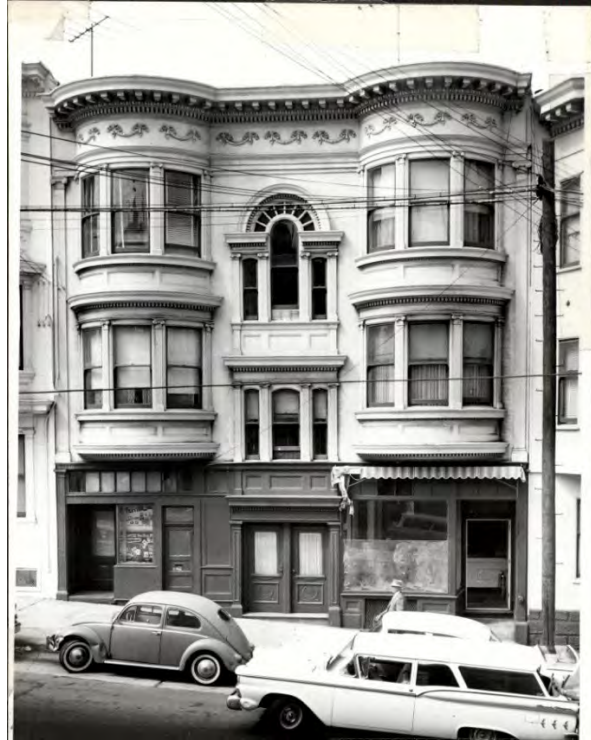
Figure 24 Enclosed Romeo flats, mixed-use building at 2035-41 Powell St. (#519), 1962, showing the use of classical moldings and proportions recalling Renaissance and Baroque Europe; Source: San Francisco Assessor's Office
