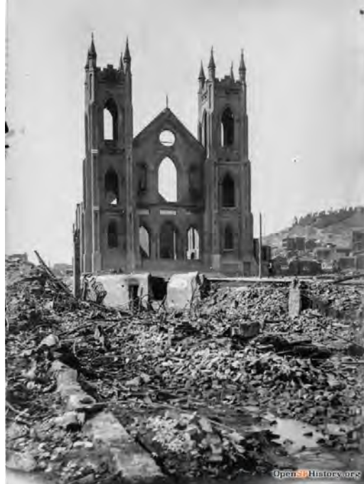
Figure 6 Surviving exterior of Saint Francis of Assisi (#683), one of the only remaining structures in North Beach after the earthquake and fire, 1906; Source: Open History wnp27.2478
